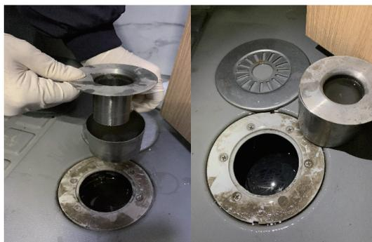
SUPPLEMENTARY FIGURE S5. The figure of the floor drains and removable water trap in a centralized quarantine apartment in Beijing.
